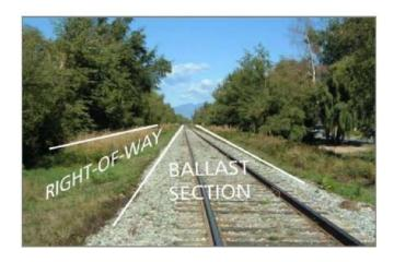
CN will use chemical control techniques on the ballast section and specific locations of the right of way throughout the network for safety reasons. Furthermore, when chemicals are applied via spray train or truck, additives called surfactants are included to make the chemical work better.
