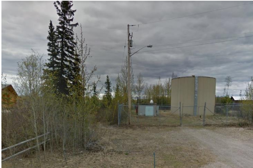
Figure 2: Gantahaz Booster Station and Reservoir
