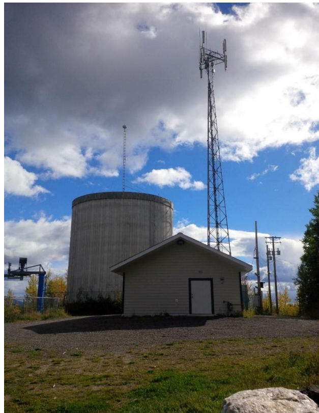
Figure 1: Town Reservoir & Booster Station
