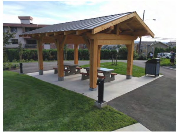
Figure 11. Shelter with Seating (City of Coquitlam, 2017).
