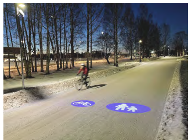
Figure 3. Wayfinding and Lane Delineation (City of Oulu, 2024).
