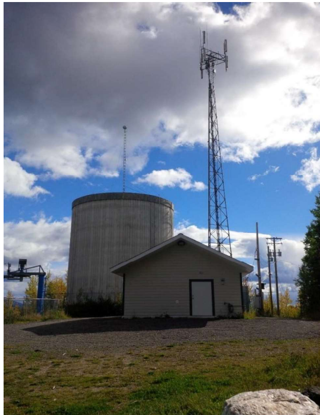
Figure 1: Town Reservoir & Booster Station
