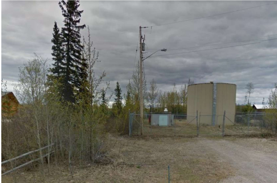
Figure 2: Gantahaz Booster Station and Reservoir
