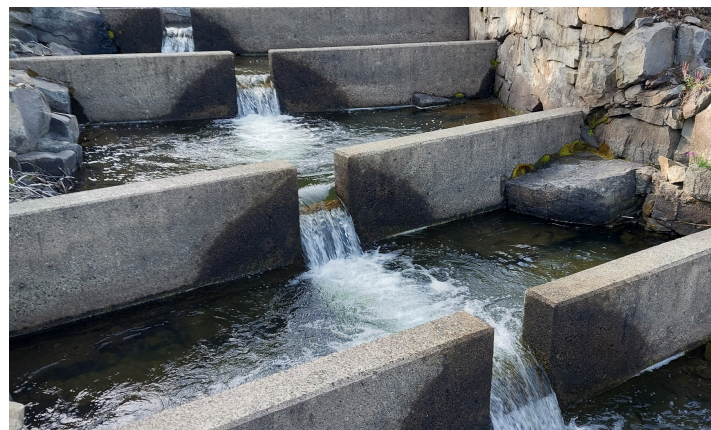
The Kemess fish ladder eases fish travel upstream to reach spawning beds.
