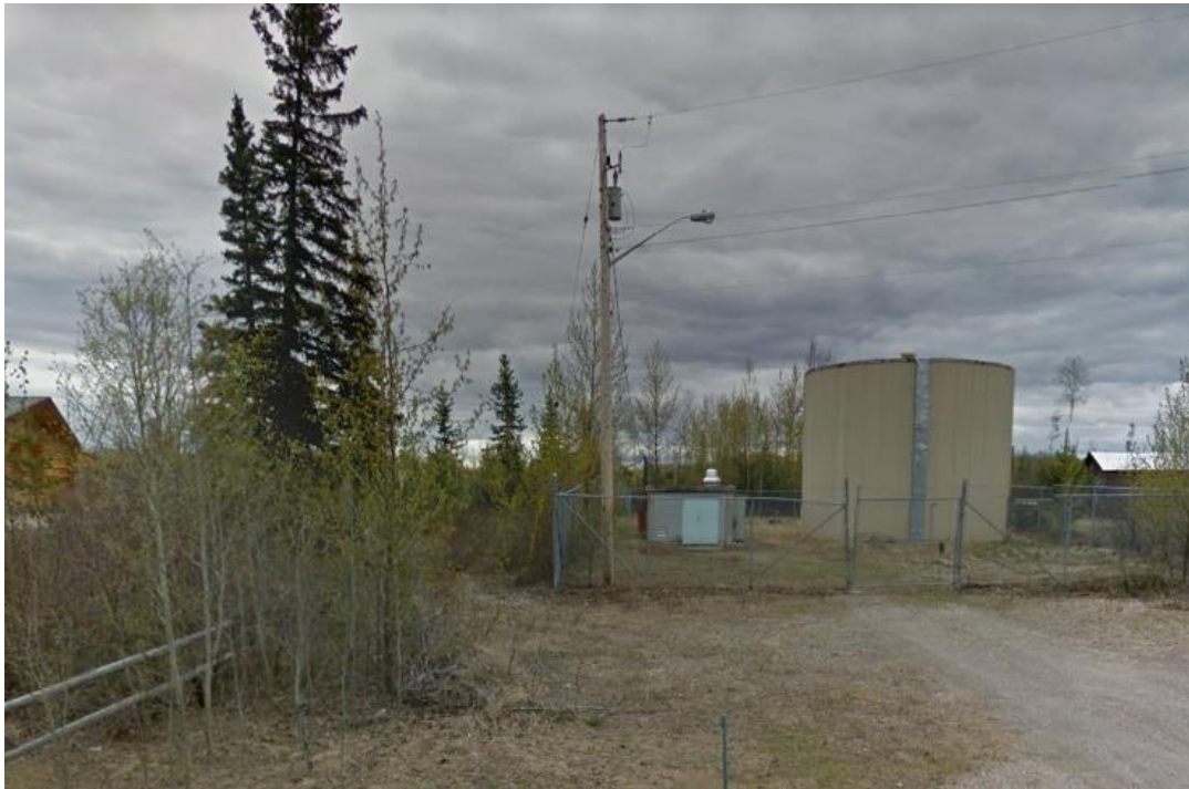
Figure 2: Gantahaz Booster Station and Reservoir
