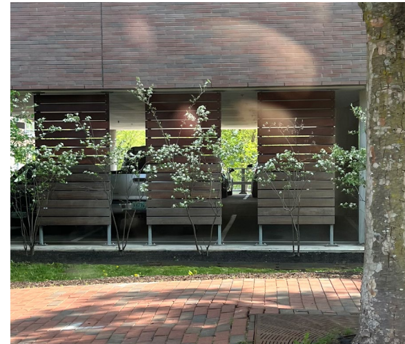
Figure 11: When provided at grade, screen or enclose parking to minimize view and impact on the public realm (3.5.j).
