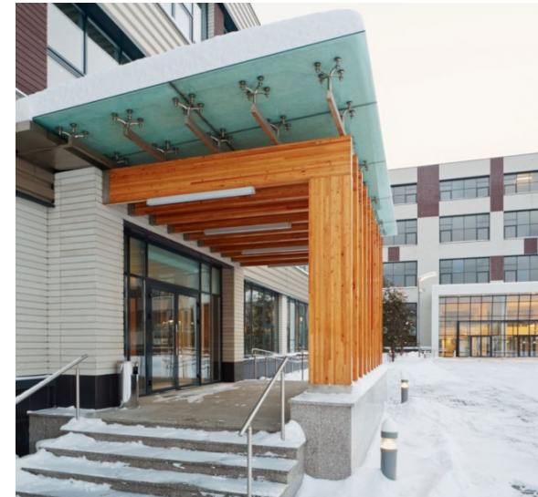
Figure 8 Incorporate snow removal and storage considerations in the design of building entries (3.4.v).
