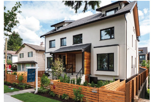
Figure 19: An example of a high-performance townhouse with a simplified building form to minimize building envelope heat loss, while also achieving many form and character objectives.
