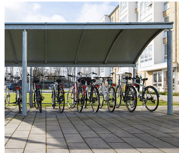
Figure 12: Covered short-term parking near primary building entrance (3.5.n).
