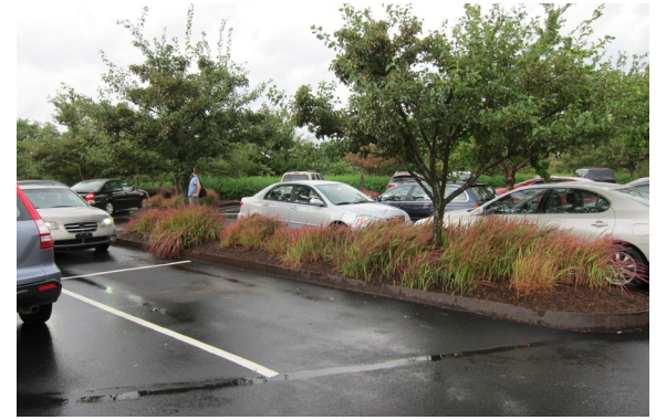
Figure 38: Provide on-site bio-retention facilities to collect, store, and filter stormwater from parking areas (6.1.h).
